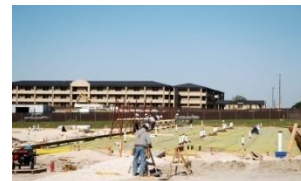
MCA Barracks Construction
